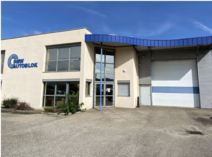
SMW-Autoblok France Headquarter, Lyon France Development, Sales, Service, Support
