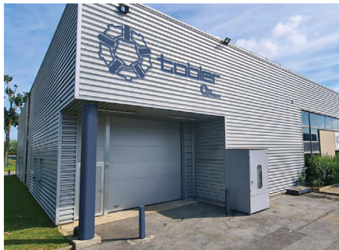
TOBLER manufacturing plant, Paris France
