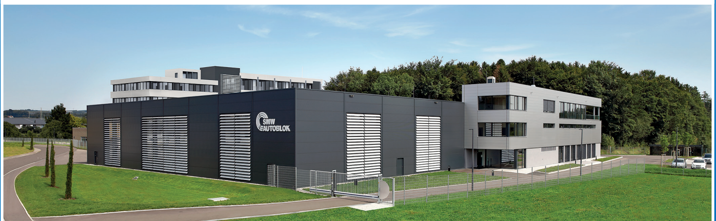
SMW-AUTOBLOK technology and logistics center Meckenbeuren
